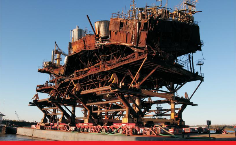
Loading and offloading offshore platforms is just about an everyday occurrance at Berard. This one however was just a little different. During one of the recent hurricanes this deck weighing 2600 tons developed a "minor" fire. Once removed from it's foundation offshore and transported to the clients facility in Gibson Louisiana, the Berard Team took action to make this final part of the move a safe and successful one.
